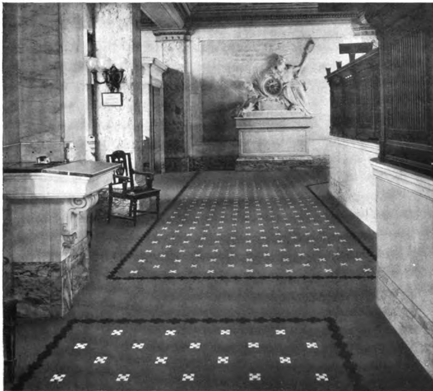
INTERLOCKING RUBBER TILING AS LAID IN THE SEABOARD NATIONAL BANK OF NEW YORK
